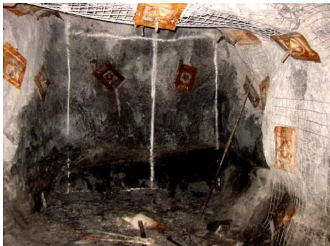
Fig. 7 Hangingwall, face and wall Threadbars in typical slot
