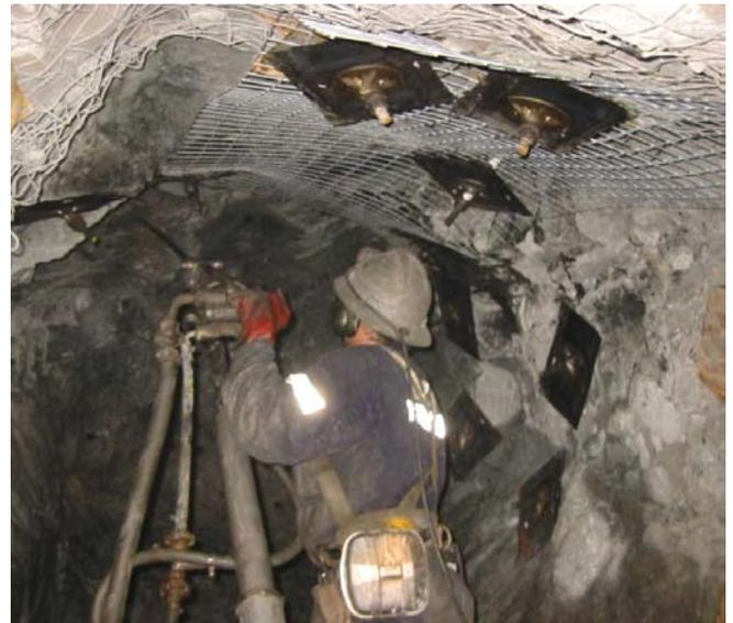
Fig. 8 Miner boring face in supported narrow slot
