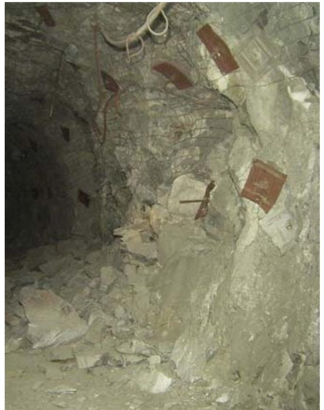
Fig. 18 Rockburst in 33N1 (porphyry), moderately controlled by support system - prior to wall meshing becoming standard in porphyry
