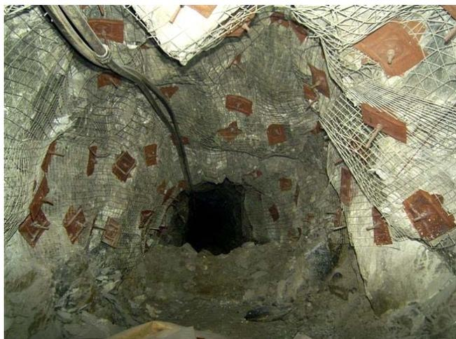
Fig. 14 Time Dependent Deformation, 35F1 Drill Drive
