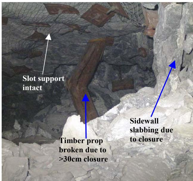
Fig. 11 Stope closure (looking down a stripped slot)
